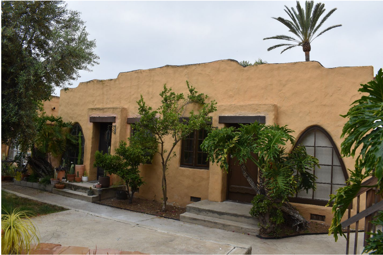
Overview of east elevation of western semi-detached, duplex style bungalow (camera facing southwest)
