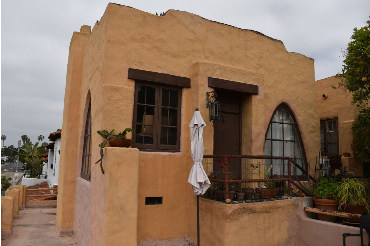
Overview of the east elevation of the westernmost detached bungalow (camera facing northwest)
